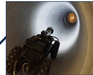
CCTV Target: Single Pipe
